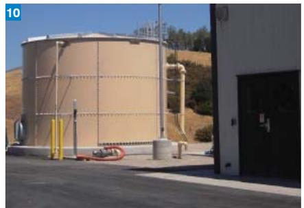
**Water desalination facility.** Chemicals are delivered to the WDTF at outdoor connections (6). Source water is pressurized through the desalination plant via these feed pumps (7). First stage EDR demineralization system (8) with the reject concentrated by the VSEP RO system (9). The concentrated brine is stored in a tank for off-haul disposal (10).
